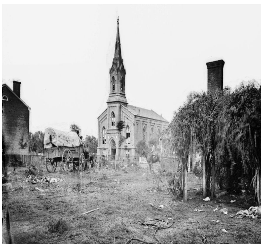
The Baptist Church in Fredericksburg, Virginia on May 20, 1864, after the city was damaged in two different major battles.
